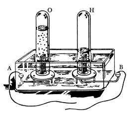
the pile; and I will take another [H] and put it over the other end [B] of the pile. And so now we have a double apparatus, with both places delivering gas. Both these jars will fill with gas. There they go, that to the right [H] filling very rapidly; the one to the left [O] filling not so rapidly; and though I have allowed some bubbles to escape, yet still the action is going on pretty regularly;
